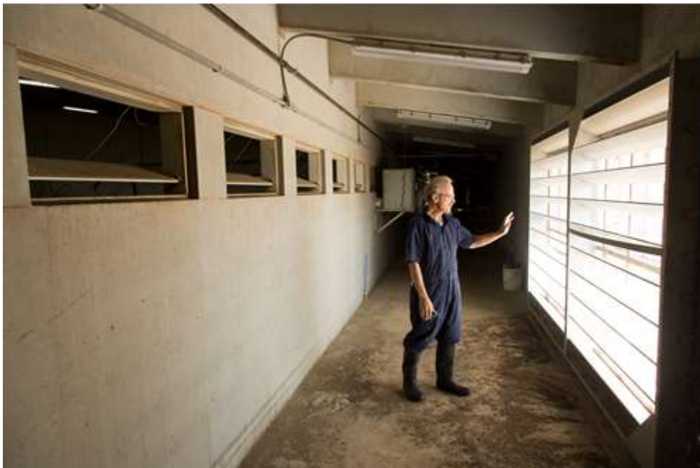
Figure 2. Exterior wall hallway that supplies inlet air to the 12 conventional rooms in the grow-finish barn.
