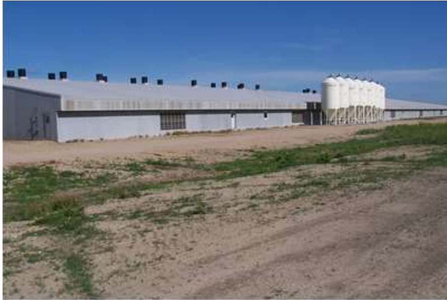
Figure 1. Outside view of 6400 head (16 rooms @ 400 pigs/room) grow-finish facilities where measurements were made comparing geothermal tempered & conventional rooms.
