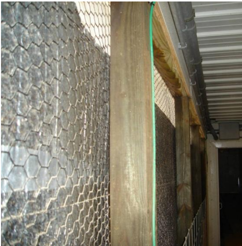
Figure 3. Bubble wrap placed on inside of curtain with aluminum side on the inside (photo courtesy of Mike Brumm)
