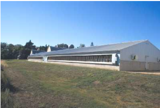
Figure 1. Typical Curtain Sided (CS) pig finishing barn.
