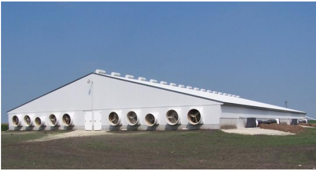
Figure 2. Common Tunnel Ventilation (TV) pig finishing barn
