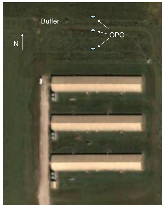
Figure 1: Photo of site.
