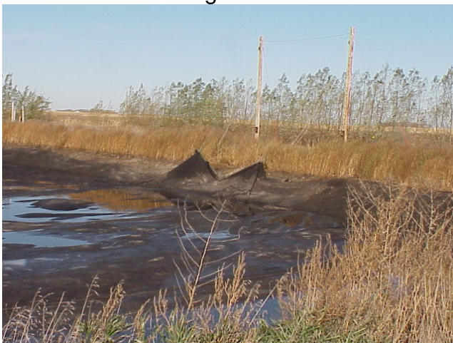
Figure 7. Geotextile cover after manure agitation and pump out
